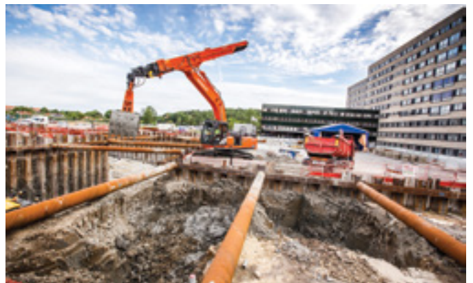
Special application excavators
