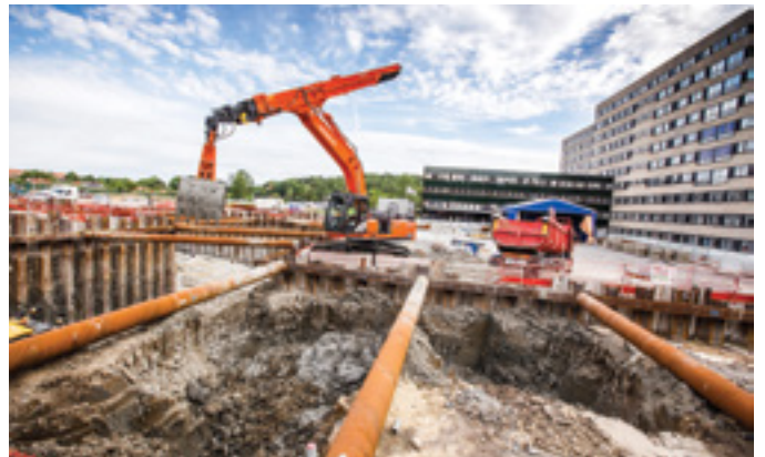
Special application excavators
